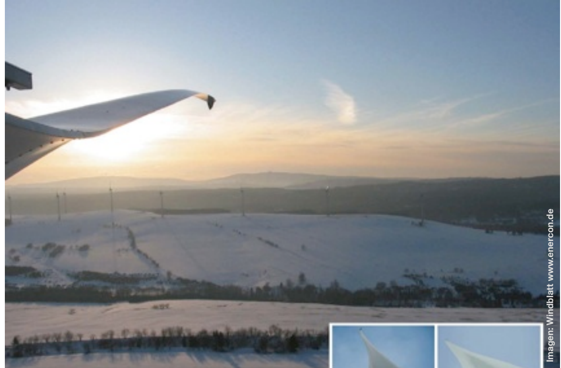
ENERCON wind farm Kryštof-Henry in the Ore Mountains.
